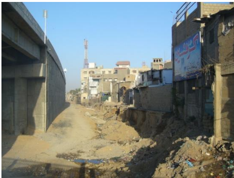
Figure-02: View of Lyari Expressway dividing a low income settlement.
