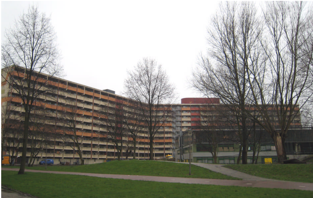
Figure 1: An example of the typical high rise buildings in Bijlmermeer.
